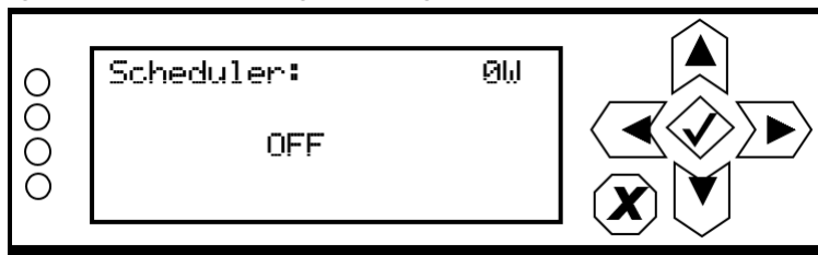
Figure 3.2.159: Enabling/disabling the scheduler - Front Panel
