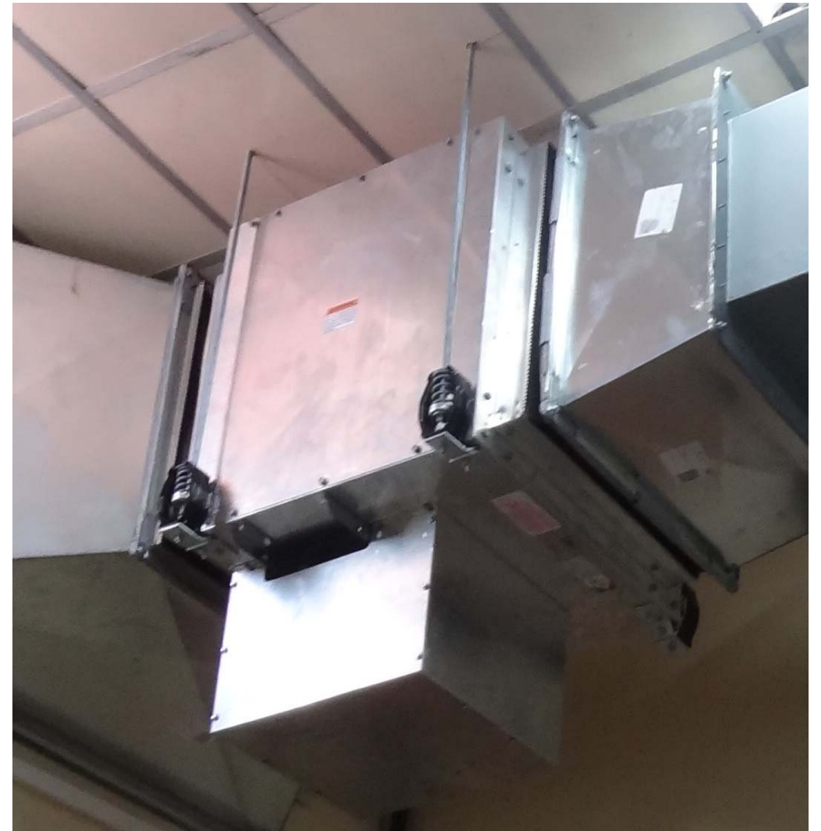
B Exhaust fan assembly (with motor at bottom orientation) U1B Mounts – Hanging Style
