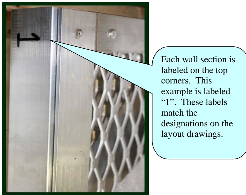
Figure 2: Example label for safety screen wall section
